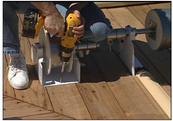
Firmly secure the independent rope reel module to the deck using all available holes.
