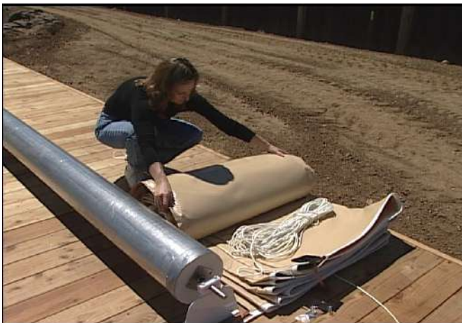
Place the cover behind the cover drum and unroll. The matte finish is on the top of the cover.
