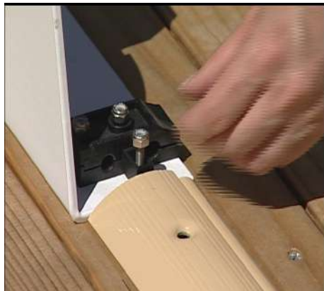
Remove the top of the track guide
