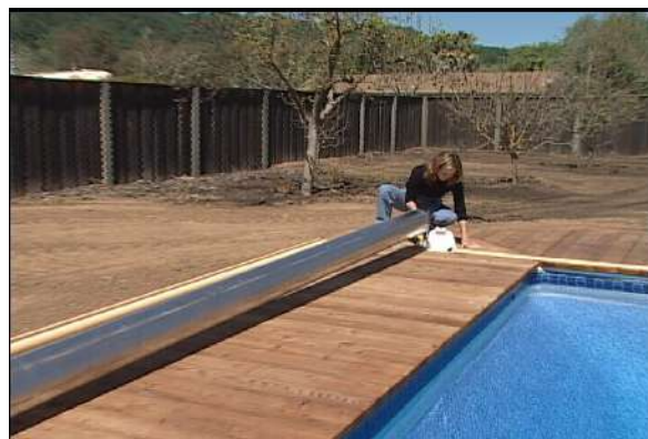
Place the shaft of each end of the drum into the U shaped section of the lower block.
