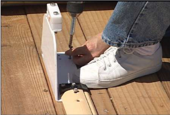
Secure back of the cover drum support with a screw.
