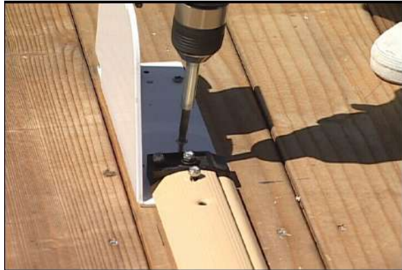
Secure front of the cover drum support with a screw.
