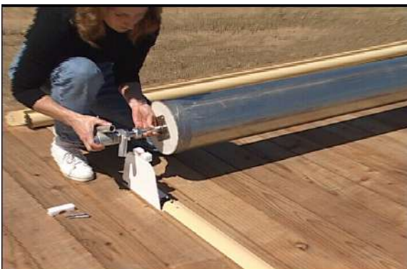
Re-secure the top half of the retaining block with the two 7/16" bolts.
