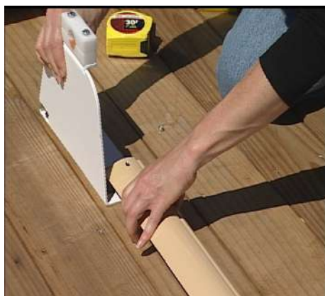
Push the track down over the stud.
