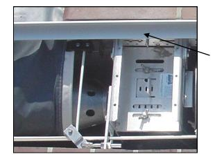
You may have to loosen and move front extrusion to gain access to the third screw & nut
