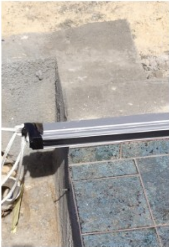
Minimum of 2" in. into vault
