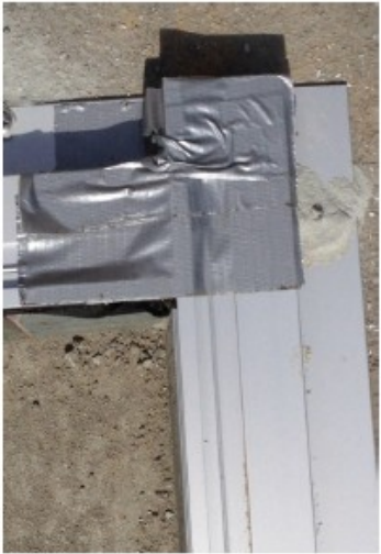
Always tape off ends and joints
