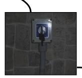
The key switch can be left attached to the Power pack and mounted to a post nearby, or relocated to a more convenient location. This can be done by "running" conduit containing four 14 ga. wires from the Power pack to the new location. There must be a complete view of the pool.
