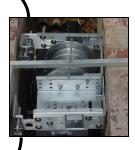
Connect the hydraulic hoses to both the Power pack and the motor unit in the vault. The hose connections do not matter at this time. Prime the system by repeatedly filling and running in one direction until you no longer need to fill the tank. If the unit is running to CLOSE while turning to OPEN, simply switch the RED and BLUE wires inside the key switch.
